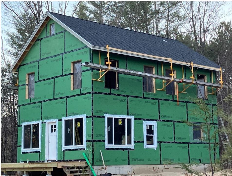
Interior being done over winter
